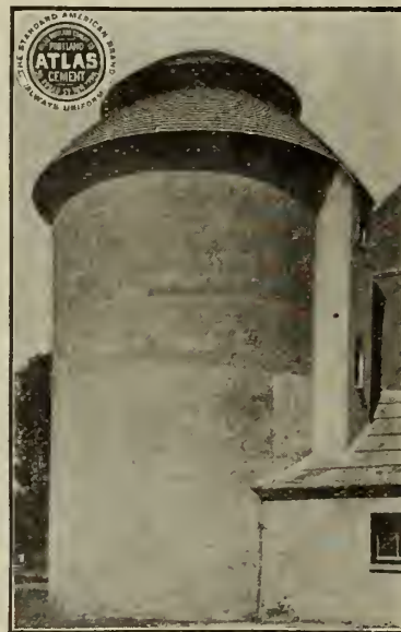
A CONCRETE SILO Gedney Farms, White Plains, N. Y.
